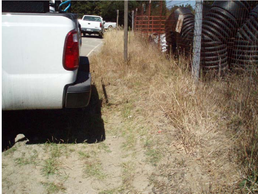
Photograph 7: Swale cleaned out.
