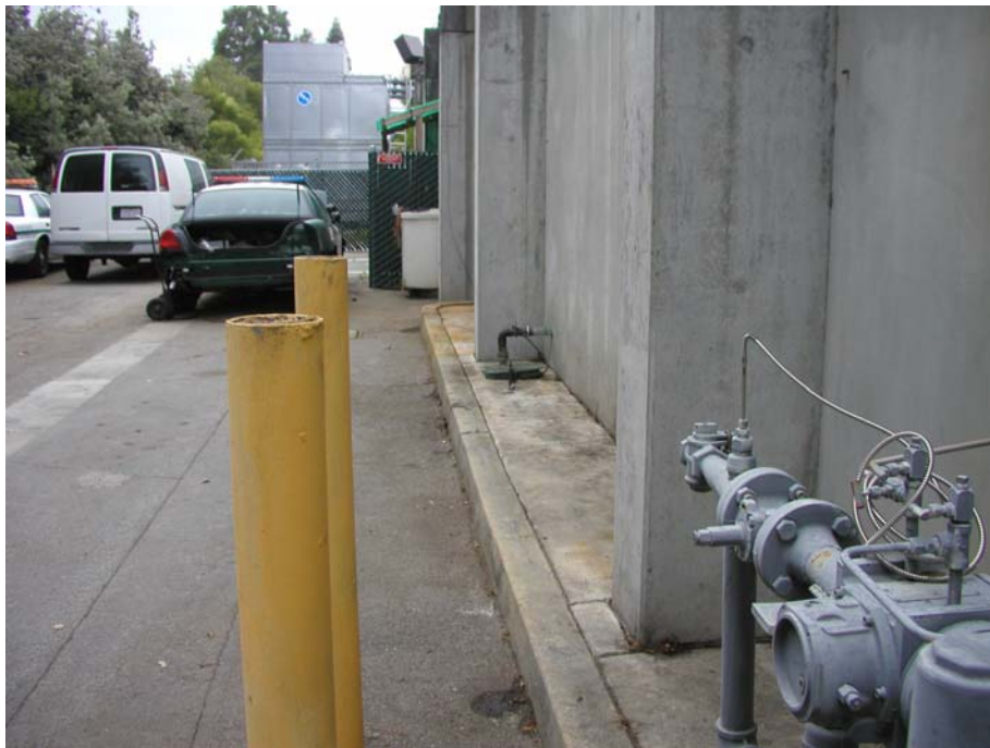
Photographs 1 and 2: Outside material storage cleaned up.
