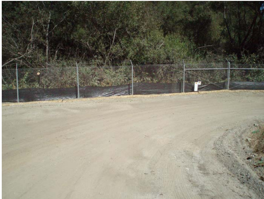
Photograph 10: Eastern boundary of maintenance yard, Rodeo Gulch riparian corridor behind fence. Perimeter controls installed.
