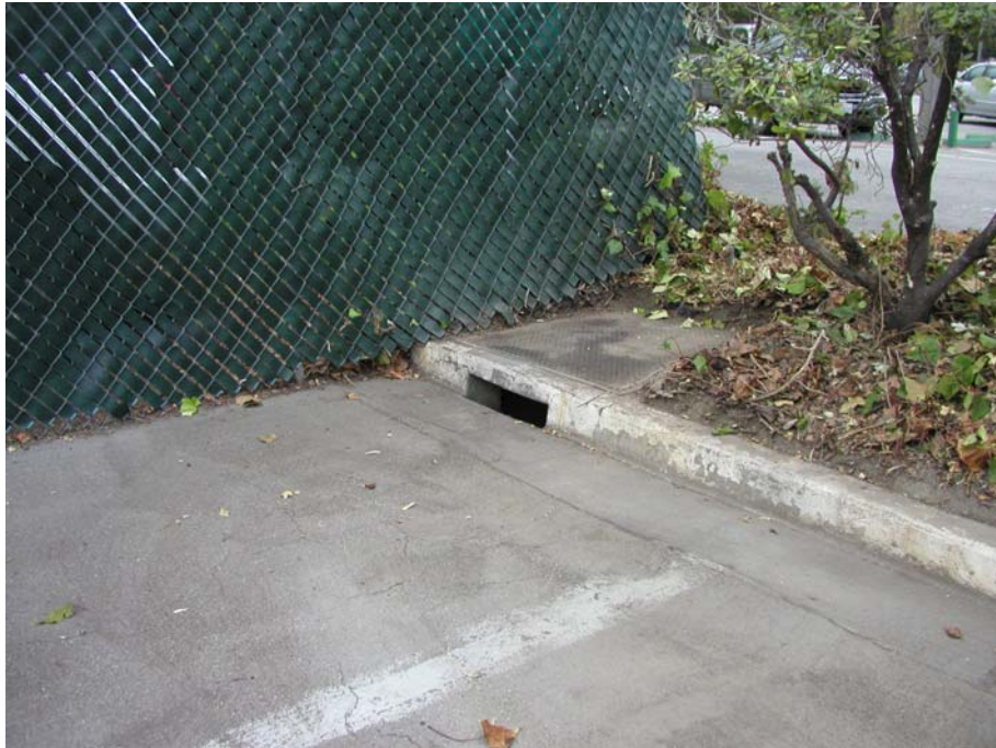
Photographs 3 and 4: Cleaned storm drain inlets.
